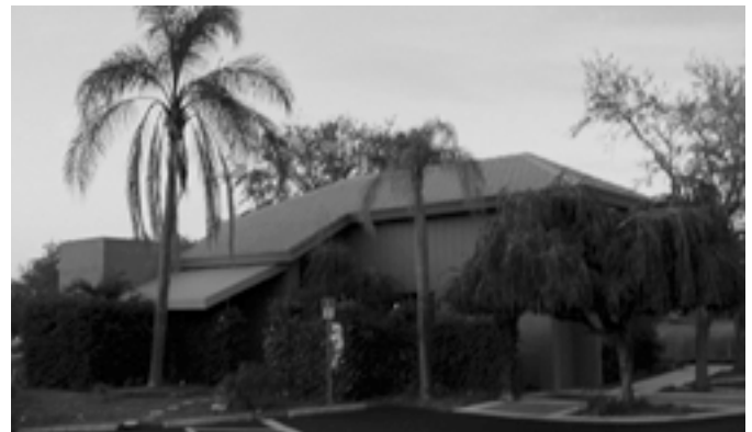
Second AAA building adjacent to headquarters along Clark Lake.
